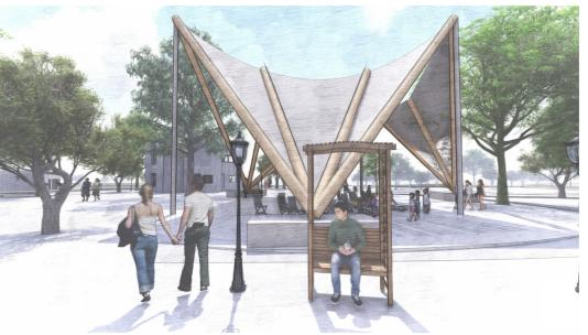
Along with being aesthetically dynamic, the pavilion has also been proven to be structurally efficient due to the capacity to cover long spans without intermediate supports.
