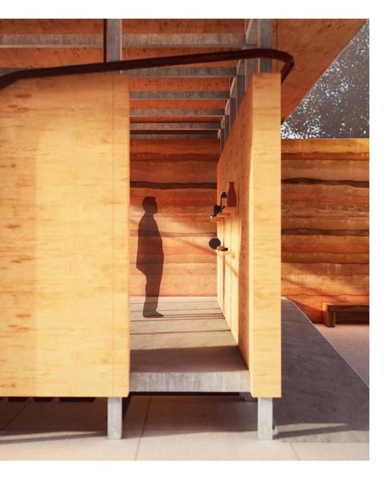
■ Earth displaced during the construction process and installation of a rainwater collection tank is reused to create layered rammed earth walls that segment the pavilion into two distinct spaces: educational + event.
