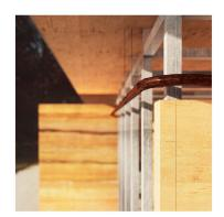
A modest approach to the structural form sees slender, hollow steel, members used as the gridded skeleton with two layered rammed earth walls which reuse the soil dug up during the construction process to reflect a physical transferring of energy from environment to architecture.
